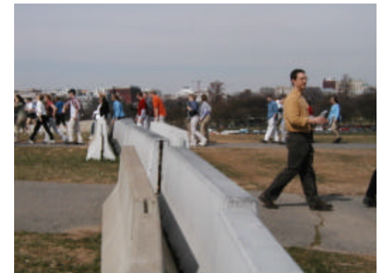
The existing temporary vehicle barrier system consists of concrete "jersey" barriers.
