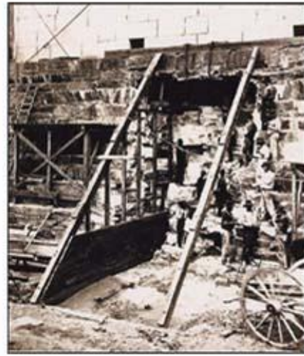
(b) Buttress Construction 1879
