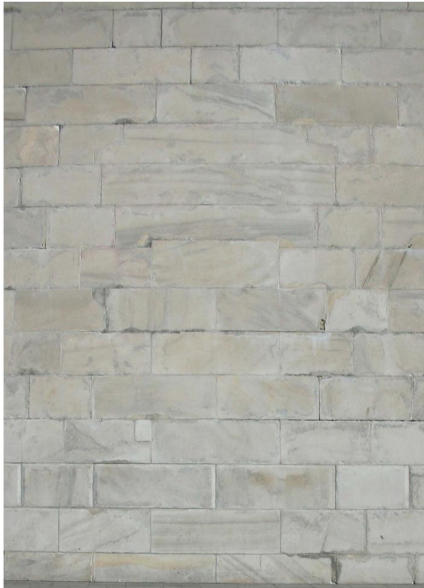
EXISTING WEST PORTAL AREA
